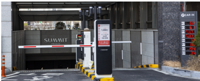
Large commercial facilities
